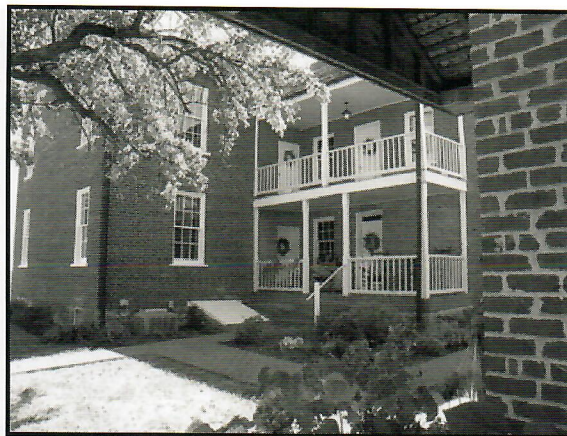
The section of Plumb Grove showing the porches was called the backbuilding.
