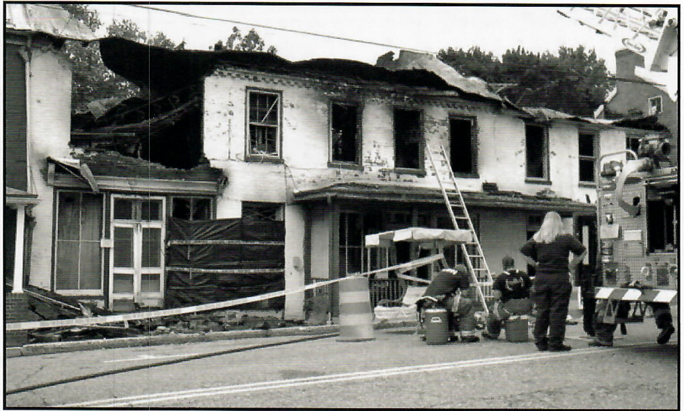
A fire during the summer of 2010 destroyed the core of downtown Clear Spring. The building on the left is 113 Cumberland Street. It was gutted from top to bottom. The large building to its right is 111 Cumberland Street. The west end section was the Brewer Hotel built around 1821. The clear spring is located next to it.
