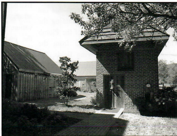
Plumb Grove outbuildings.
