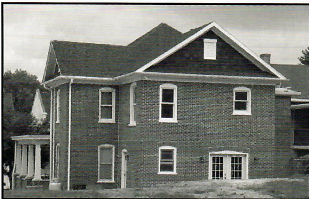
Above view shows new back addition at 10 Cumberland Street. Jim Snyder did a fantastic design of having his new addition blend with the rest of the house. The construction work was done by Mark Myers. The photo on the right shows the house as it neared completion in the early 20th-century.
