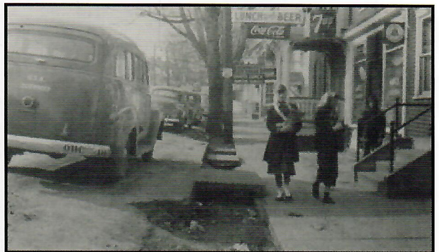
Cumberland Street in Clear Spring as it appeared during the early 1950’s.
