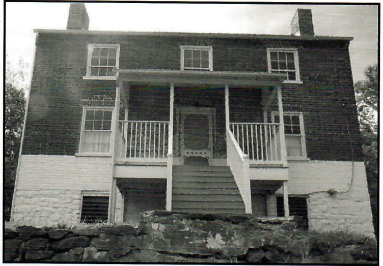
Lockhouse 49 is located at Four Locks, Maryland.
